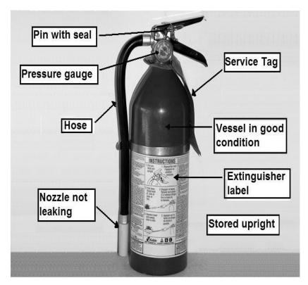
Pin with seal – the pin should be held in place with a plastic seal. The seal must be broken to remove the pin. Watch for long pins, as they may be bent and difficult or impossible to remove.
