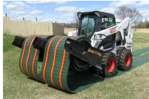
Note this skid-steer is laying turf protection.
